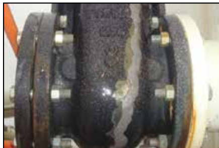
Valve leakage plugged with ARC 5ES.
