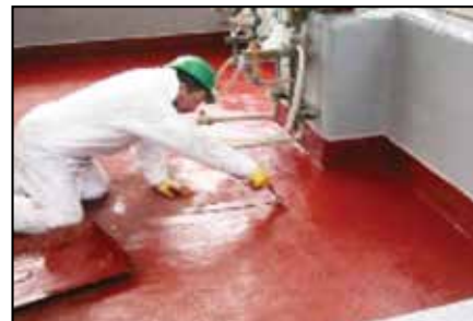
Applying ARC CS4 topcoat.
