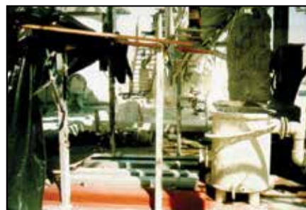
ARC 988-coated processing areas.
