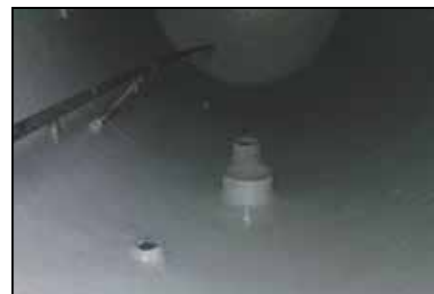
Coated tank internals.
