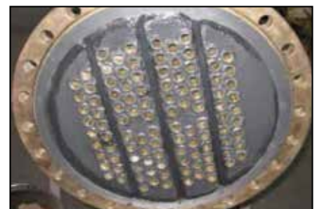
Completed tube sheet.
