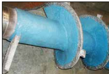
ARC MX1 applied and tips welded.
