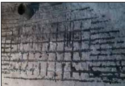
Chest wall after tile removed and blasted.
