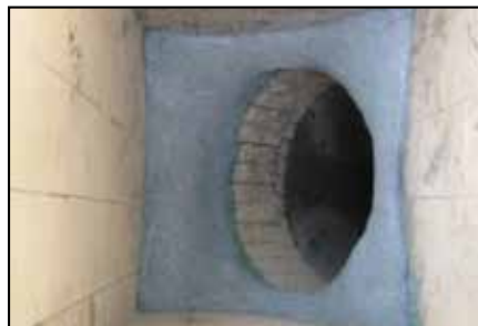
Installation of ARC MX5.
