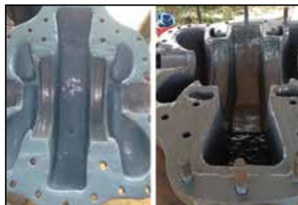
Repair being performed, body and cover.
