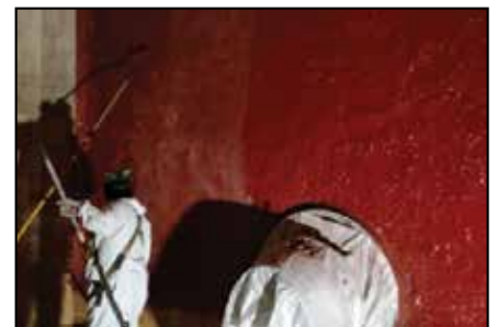
Applying NVE sealer coat.
