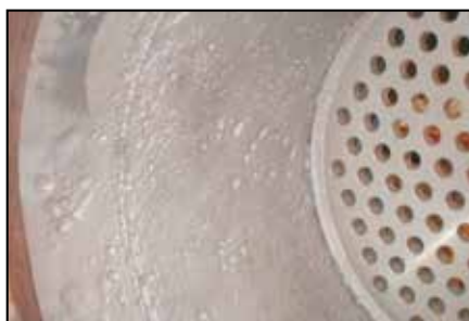
After cleaning and decontamination, ARC 858 is applied to fill and smooth surface.
