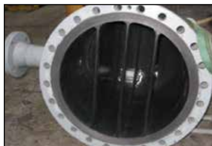
Repaired divider plates.
