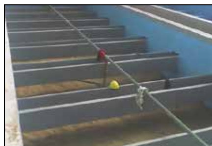
Installing ARC S1PW coating.
