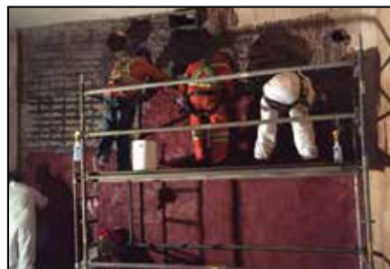
Installing ARC NVE coating.
