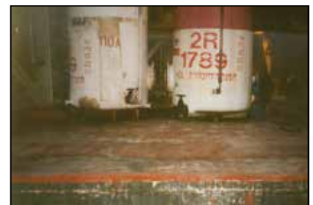
ARC 988-coated floor areas.
