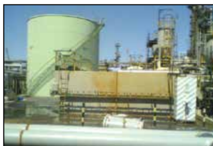
Basin in petrochemical complex.
