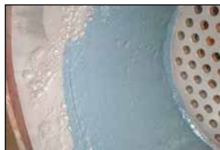
After application of ARC 858, ARC SD4i is applied for protection and enhanced flow efficiency.
