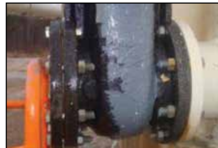
Repaired valve with ARC 5.
