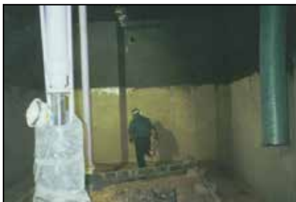
Concrete protected with ARC 791 and ARC 988.
