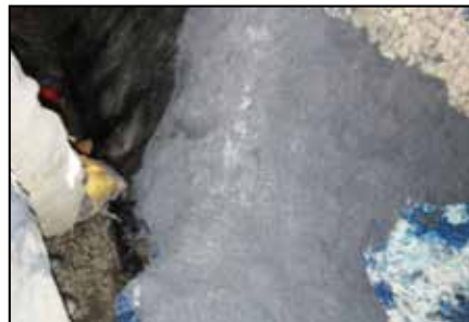
Applying ARC I BX1.
