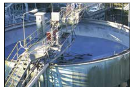
ARC S2 still in excellent condition.
