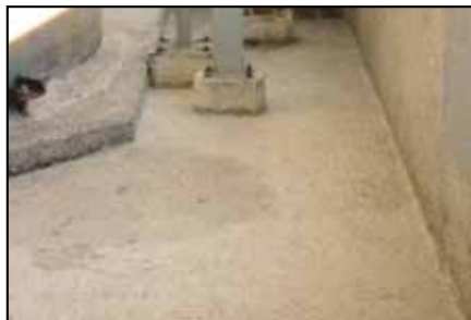
Cleaned and prepared surface.
